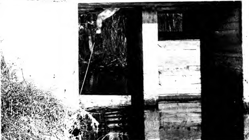
Peter Stearns lifts the last plank out of the flume to release the winter flood.
